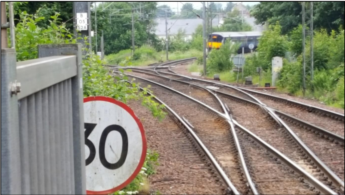
Photo: Westerton Junction, showing a train leaving on the single track, having crossed the double line. (Credit: David Prescott)
